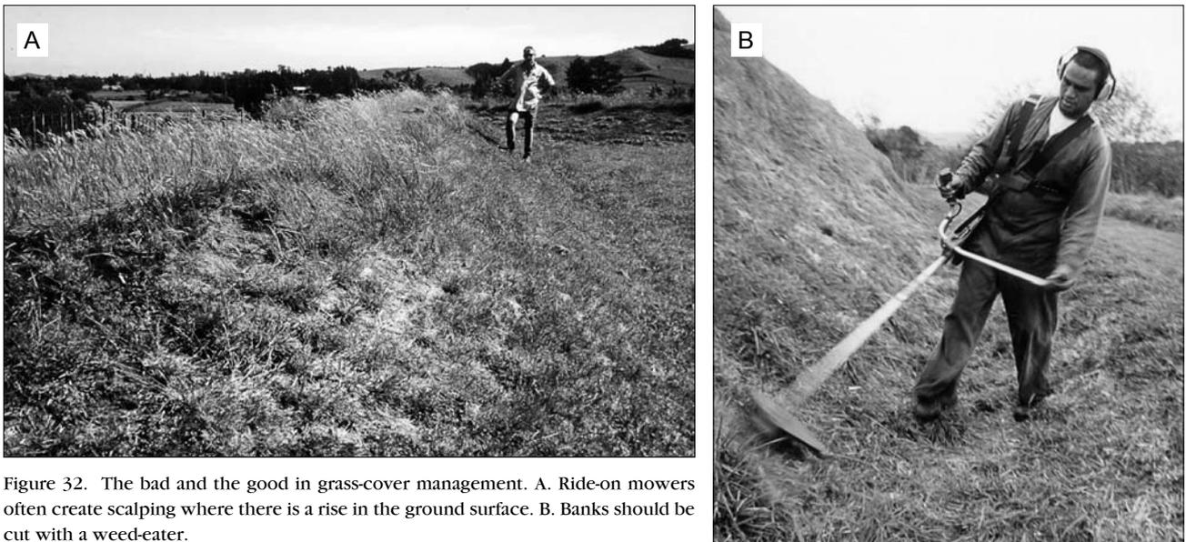
Figure 32. The bad and the good in grass-cover management. A. Ride-on mowers often create scalping where there is a rise in the ground surface. B. Banks should be cut with a weed-eater.
